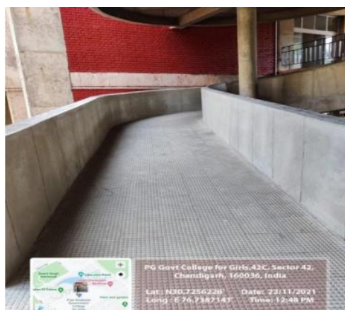
Ramp in Main Building
